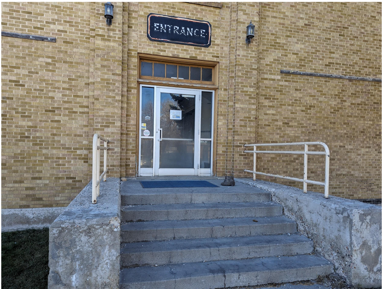
Entrance on Center Street, now considered the front of the building.
